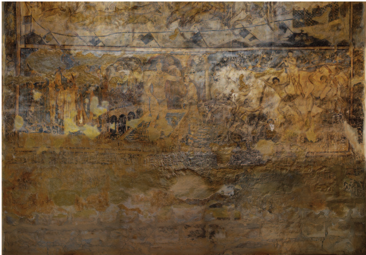
Qusayr 'Amra. Basílica Hall West Wall Internal Elevation. Scale 1/25. November 2009 Spanish Archaeological Mission/ Institute Juan de Herrera Survey Director: Dr. Ignacio Arce. Photo Rectification: Mr. Ignacio Moscoso.
